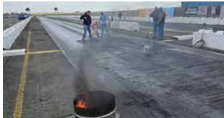
Workers do track prep at the starting line.
